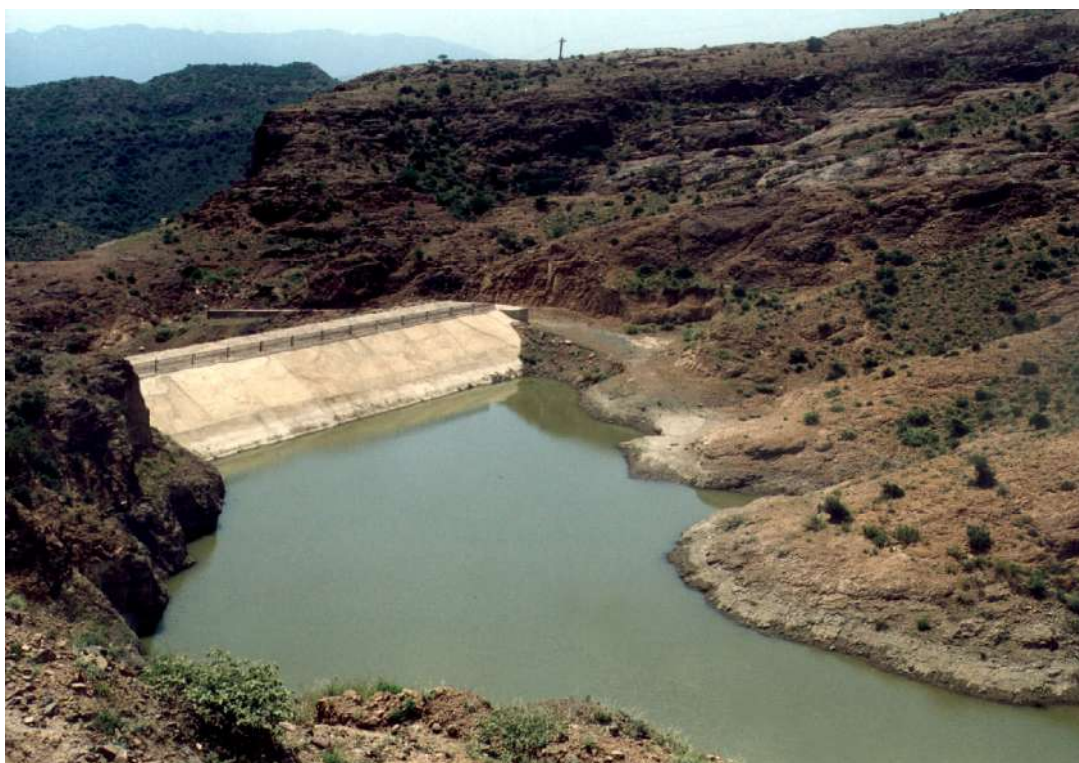
Figure 5-2: Typical small dam in the mountain regions in Yemen
